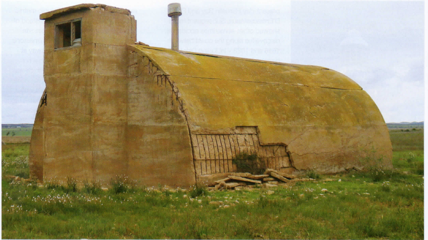
The remains of Number 203 Cowell Radar Station.
